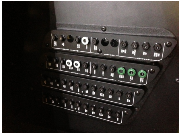
Image 18: Circuit Breaker Panel Co-Pilots Side
