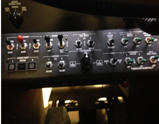
Image 20: Lower Switch Panel Pilots Side 1
