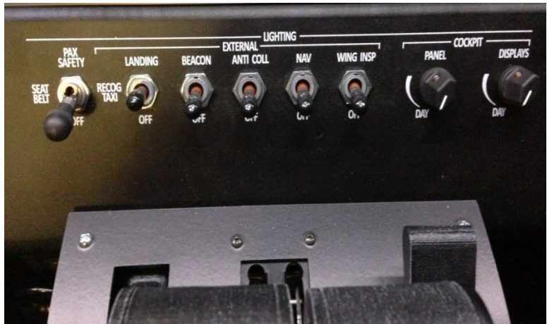
Image 25: Lower Switch Panel Center
