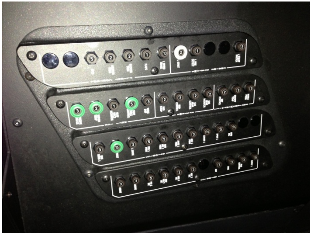
Image 17: Circuit Breaker Panel Pilots Side
